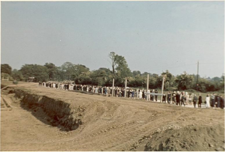
Turning of the sod – guests viewing Science Building site
